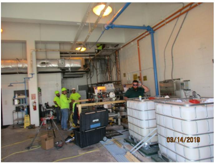
• Scaffolding needs to be Red Tagged. It is missing fall protection, proper planking, toe boards and proper access. 1926.451-453
